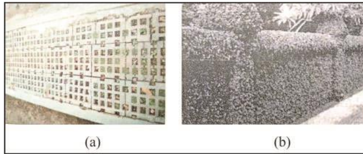
Figure 2. (a) Grass block to prevent flooding, (b) Hedgerows to reduce noise (Source: (a) Karyono, T. H., 2010, (b) Christina, E. M., 2013)
