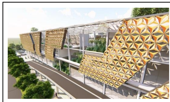
Figure 7. Metal secondary skin as a buffer
