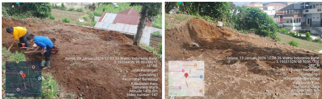
Figure 2. Land conditions during land preparation.
