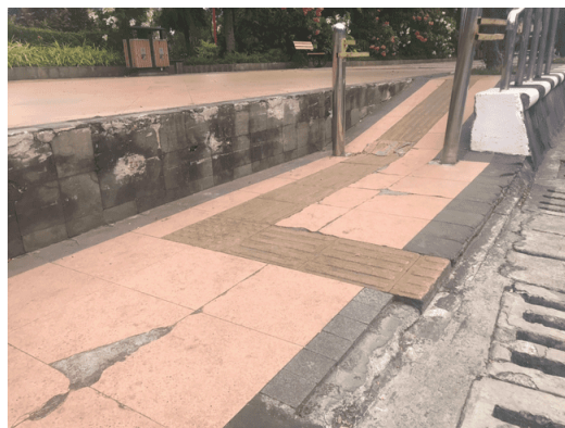
Figure 5. Floor damage at Jalan A Yani Entrance Source : author document, 2024
