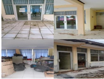
Figure 4.2 Condition of UPTD P2PMKS Nilam Suri
